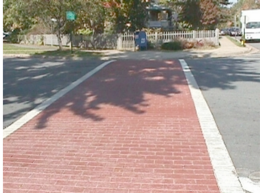
Example of textured crosswalk, which is highly visible to both pedestrians and vehicular traffic
